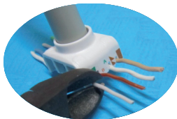
Figure 2b - Trim wires so they are level with cap
